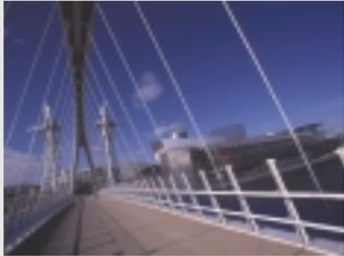
Ahead of you is the impressive Lowry footbridge. The lifting footbridge spans the Manchester Ship Canal linking The Plaza with Trafford. Opened on 28 April 2000, at 92 metres long the single span bridge provides pedestrian and cycle access across the canal while continuing to maintain access for occasional shipping traffic.
